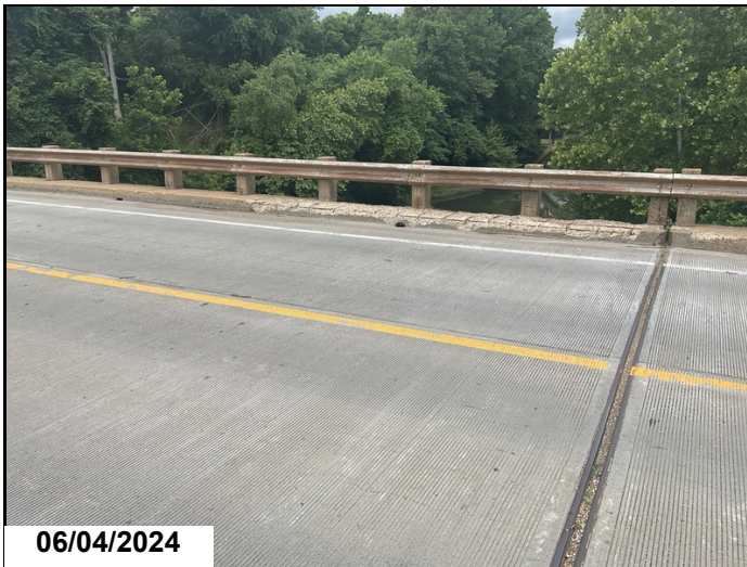
Left curb in span #3 showing spalling with exposed rebar.
