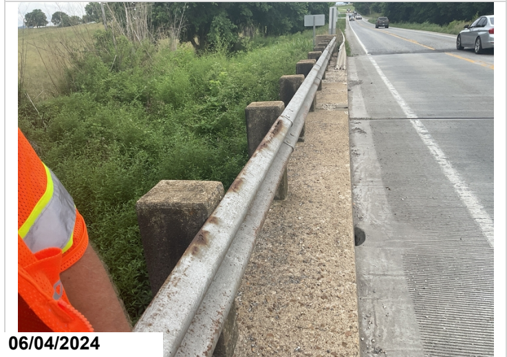
Cs3 corrosion on the right railing in span #2.
