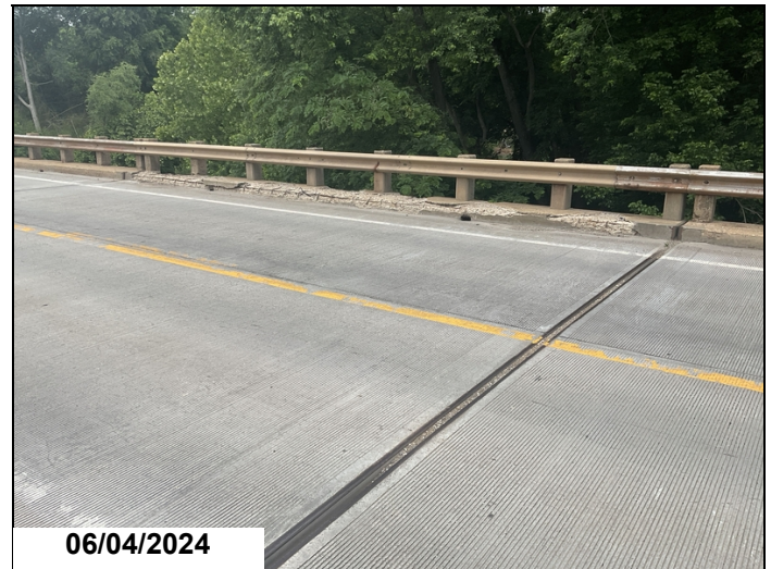
Left curb in span #6 showing spalling with exposed rebar.
