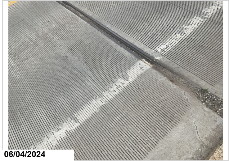
12' of deck cracking at the end of span #1.
