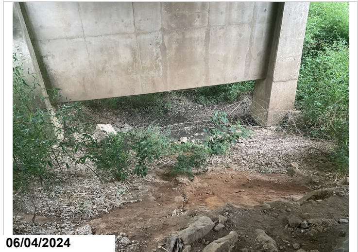
Local scour around the bent #1 columns with embankment erosion at the toe of the abutment #1 slope.
