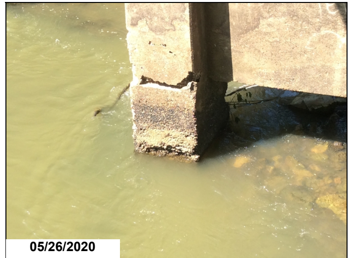
Bent 3 column 2 ahead side side large areas of spalling with steel exposed.
