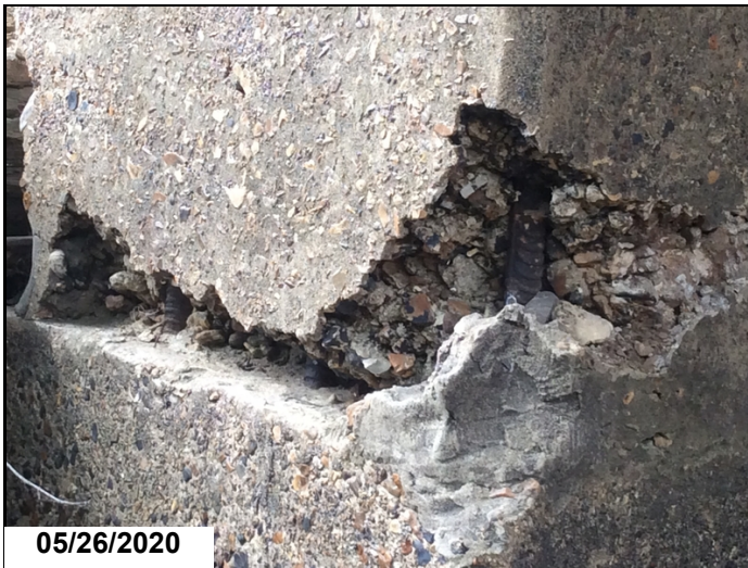
Bent 3 ahead side of right column 2 steel exposed.
