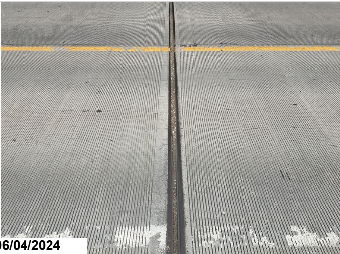
Strip seal condition over the bents. Loose debris impactation typical.
